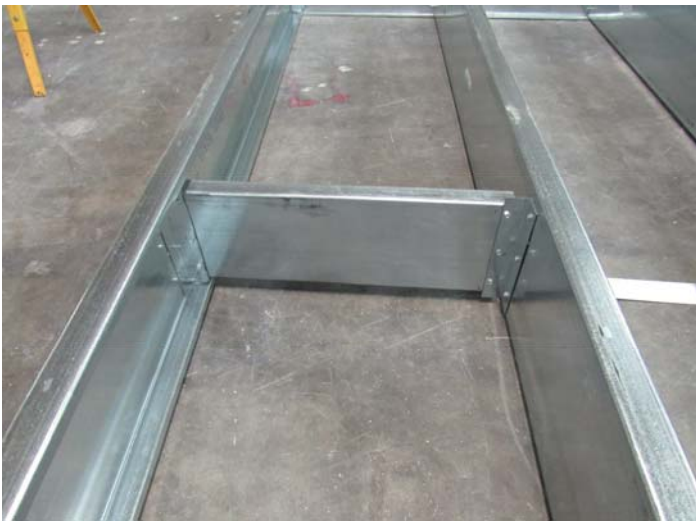
End Blocking Connection
