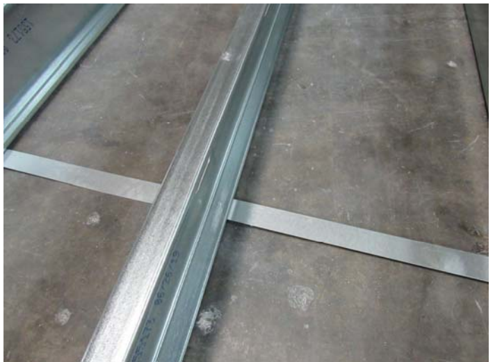
Strap Bracing Connection
